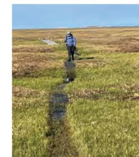
RIGHT: USE OF RUBBER MATS TO CREATE PATHS THAT PROTECT THE GROUND - TRANSITORY BOARDWALK
